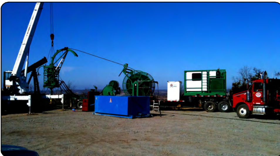
Complete cleanout setup including CT unit, pump truck, and flowback tank.
